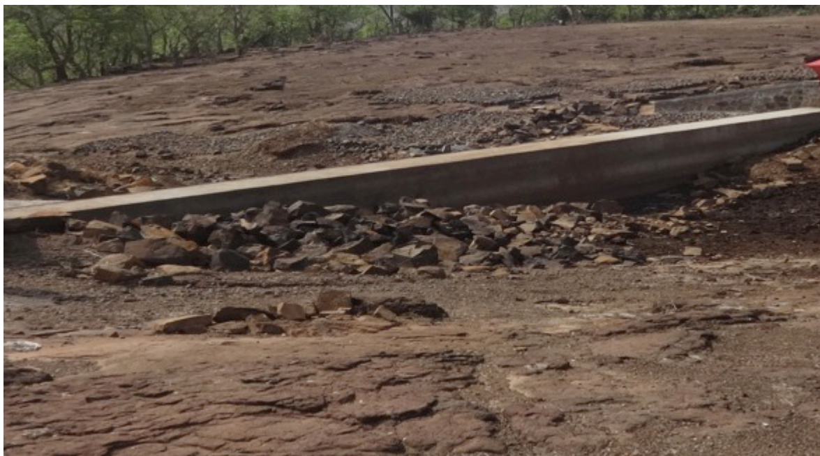
Figure 11 Siltation in bund in Kurlod habitation
