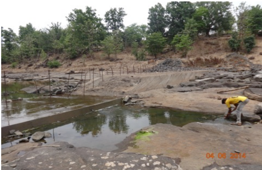
Figure 8 Incomplete bund at Manipada (Kurlod)
